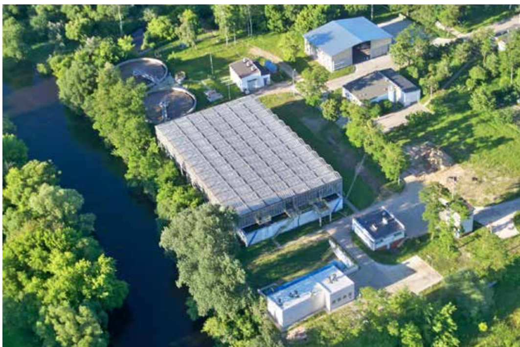
Sewage treatment plant in Sochaczew. Photo ZWiK Sochaczew Sp. z o.o.
