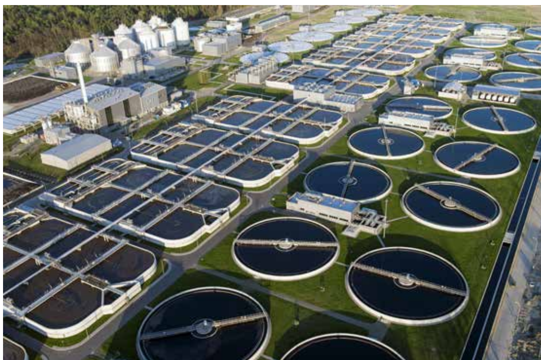
Sewage Treatment Plant "Czajka" in Warsaw. Photo Kacper Kowalski for the Urban Water and Sewage Company
