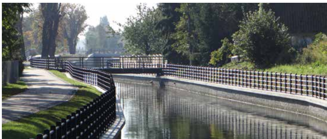
Radunia Channel in Gdańsk modernized after the flood. Photo Lech Makara
