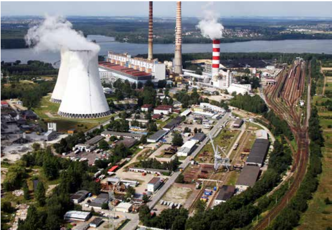
With the resources of NFEPPM, during 25 years, the largest Polish power plants were modernized. Photo NFEPPM archives
