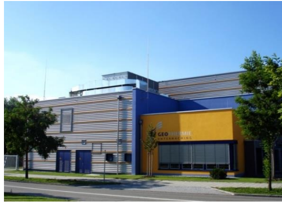
Unterhaching Geothermal cogeneration plant
