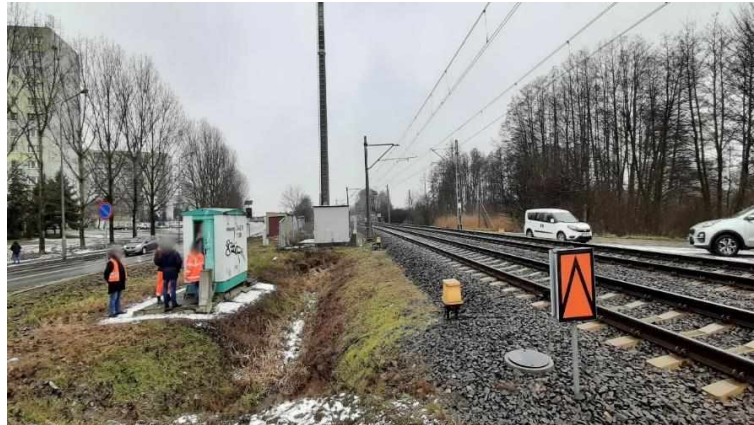
Photograph 5 – A view of track no. 2 from the road from the distance of 5 metres from the outermost rail (own material of PKBWK)
