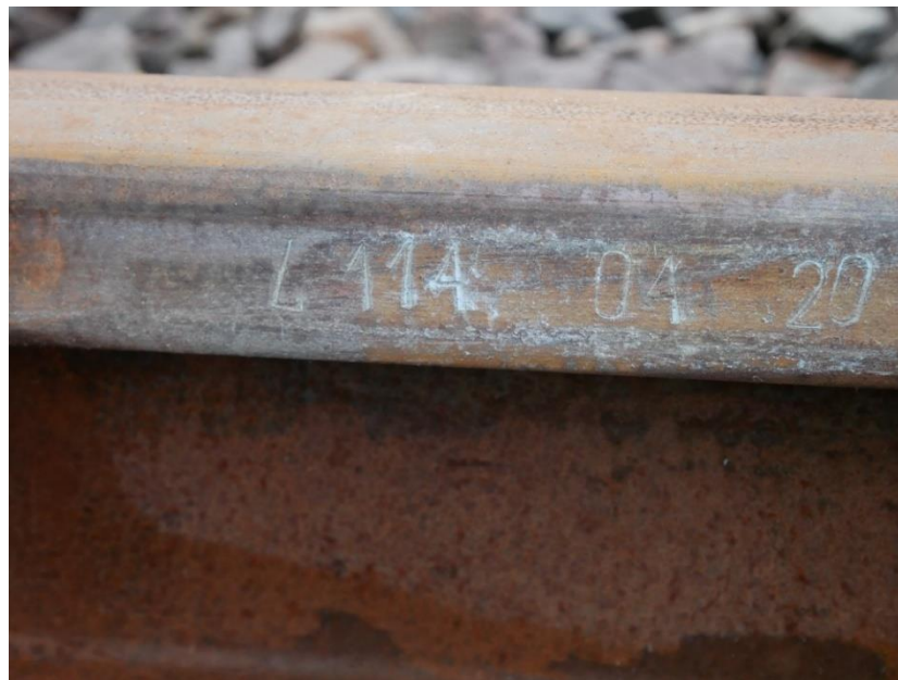
Photograph 6 – Welder operator identification number
