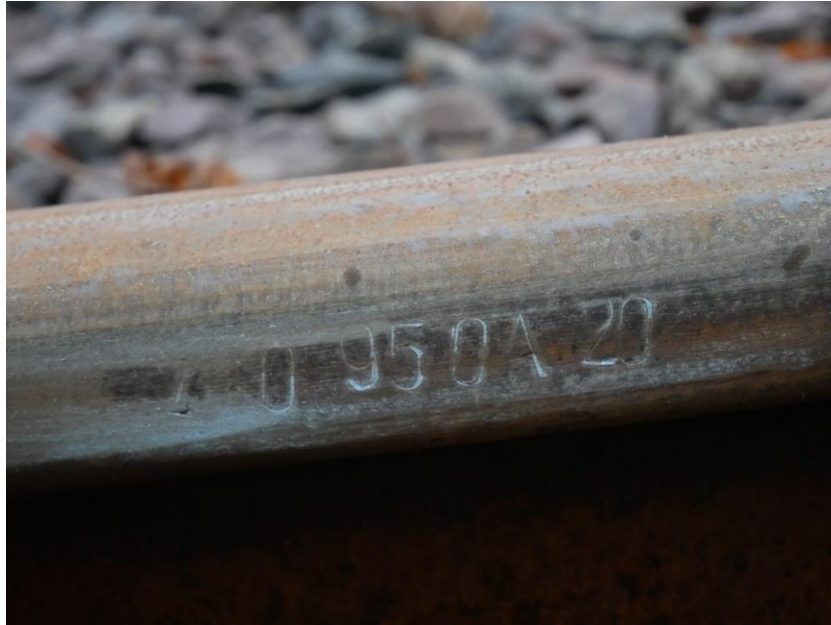
Photograph 7 – Welder operator identification number
