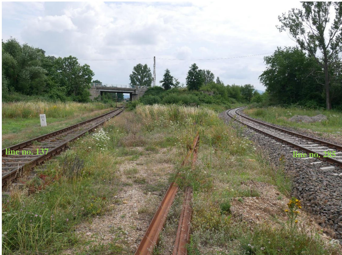
Photograph 8 – View of the collision site on line 285 (right) adjacent to active line 137 (left)
