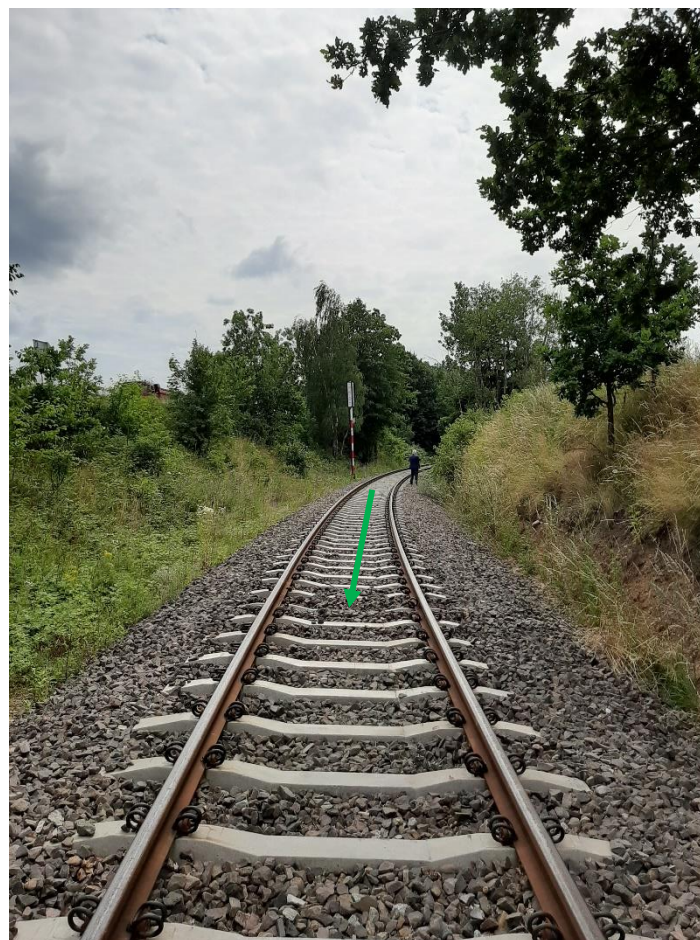
Photograph 5 - View towards the entrance semaphore (Source: phot. SCRAI)
