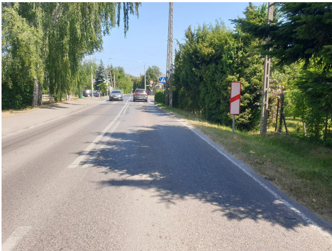
Photograph 12 – Visibility of the level crossing from 60 m (source: PKBWK own material)
