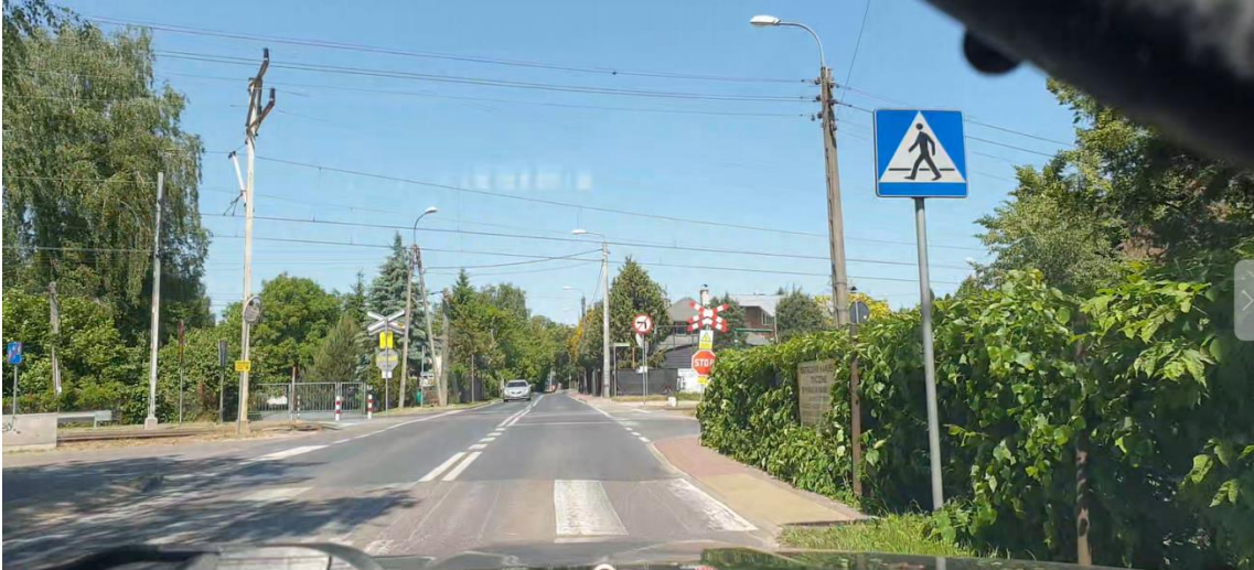
Photograph 14– Visibility of the level crossing from 30 m (source: PKBWK own material)
