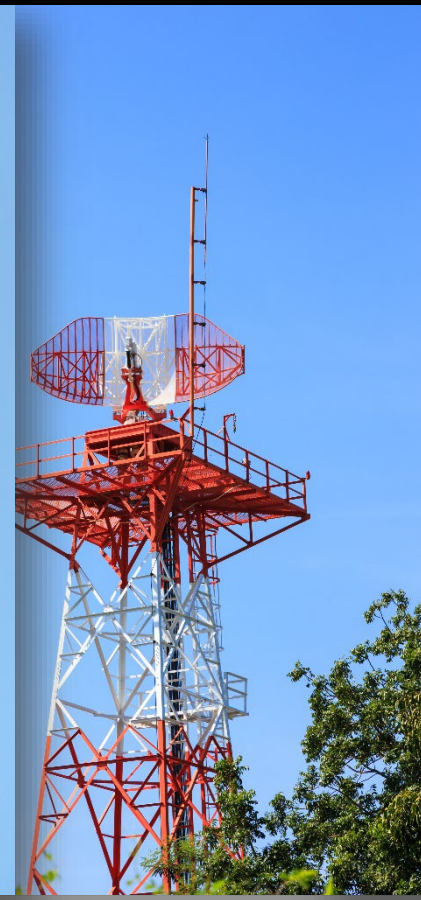
radar systems and satellite earth stations
