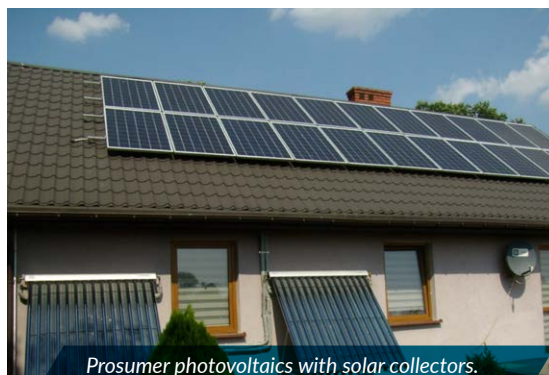
Prosumer photovoltaics with solar collectors. Photo: Agricultural Advisory Centre in Brwinów, Radom Branch.
