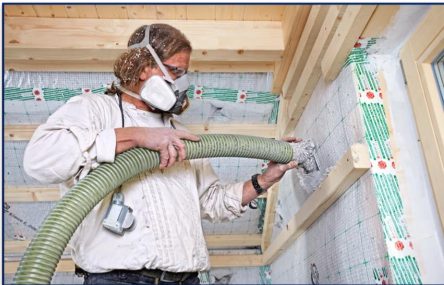
fot. 3 onet.pl: blowing in the cellulose fibres
