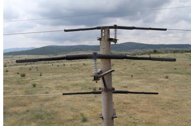
200 km of overhead power lines will be secured by protective insulations
