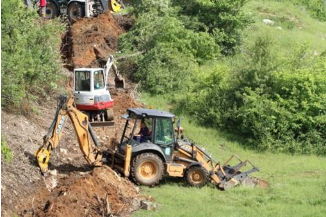
52 km of overhead power lines will be installed underground
