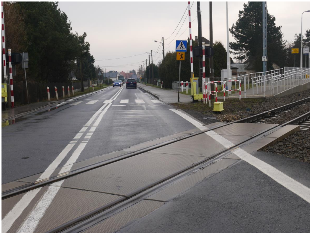
Photograph 4 - A general view of the occurrence site (evidence material of PKBWK)
