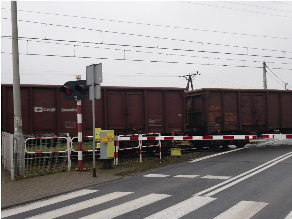
Photograph 6 – Position of the pedestrian crossing
