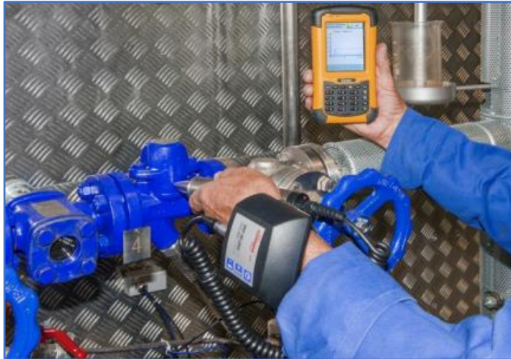
Pic. 4 Krzysztof Szatucki: ultrasounds used to control a trap
