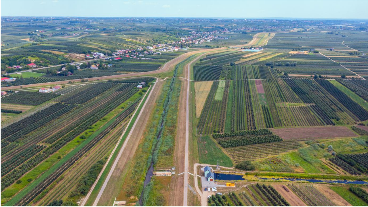
Photo 10. Subtask 4 - Modernised embankments of the Koprzywianka River – bird's eye view (source: SWH PW's own materials).
