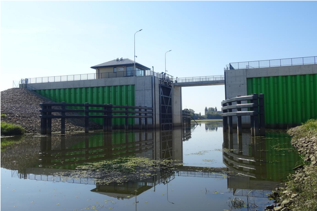
Photo 9. Subtask 3 - Implemented construction of the flood gate in Sandomierz – general view (source: SWH PW's own materials).
