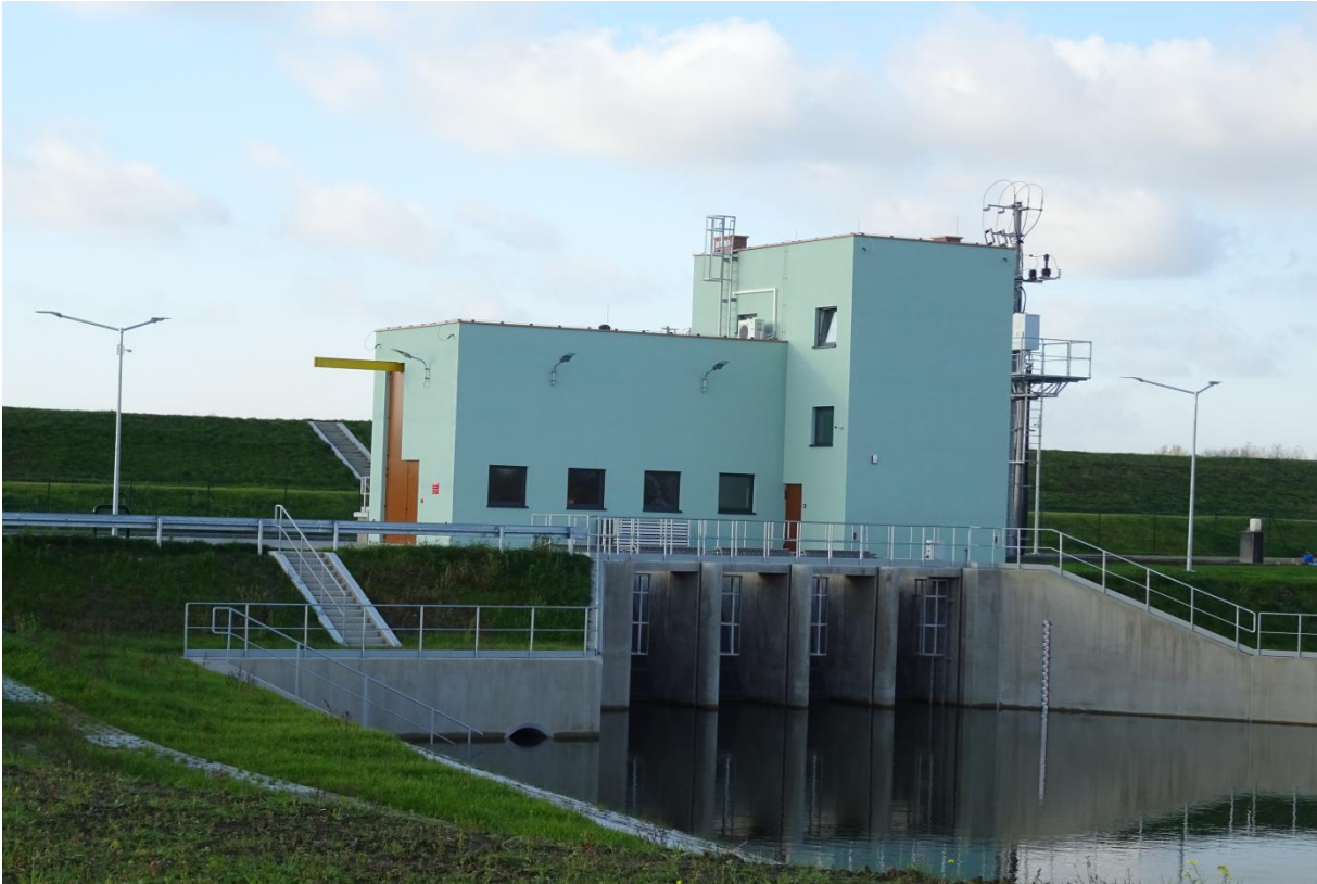
Photo 6. Subtask 1 - Implemented construction of the pumping station in the town of Koćmierzów – general view (source: SWH PW's own materials).
