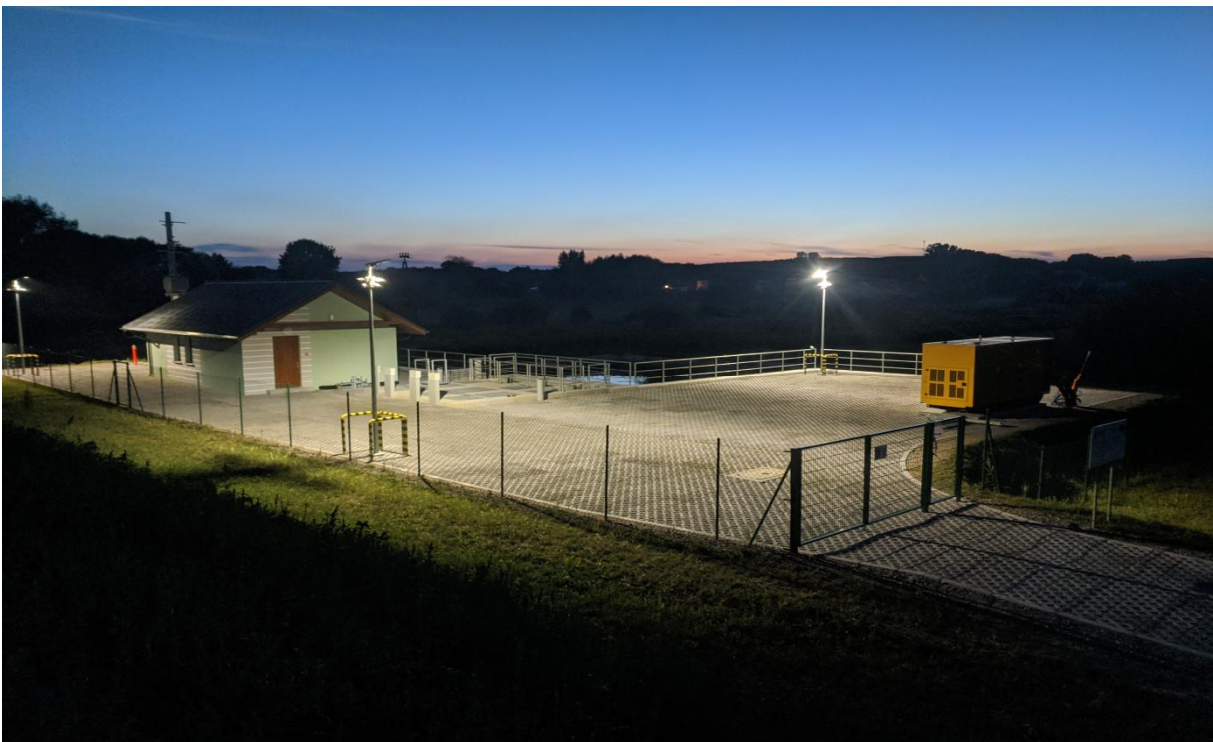
Photo 11. Subtask 5 - Implemented construction of the pumping station in the town of Szewce – general view (source: SWH PW's own materials).
