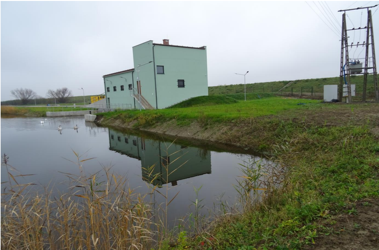
Photo 7. Subtask 2 - Implemented construction of the Nadbrzezie pumping station – general view (source: SWH PW's own materials).
