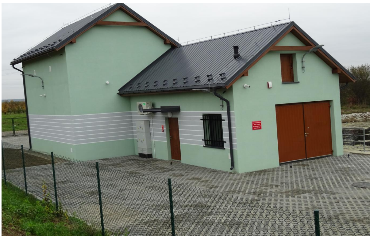
Photo 12. Subtask 6 - Implemented construction of the pumping station building in the town of Zajeziorsze – general view (source: SWH PW's own materials).
