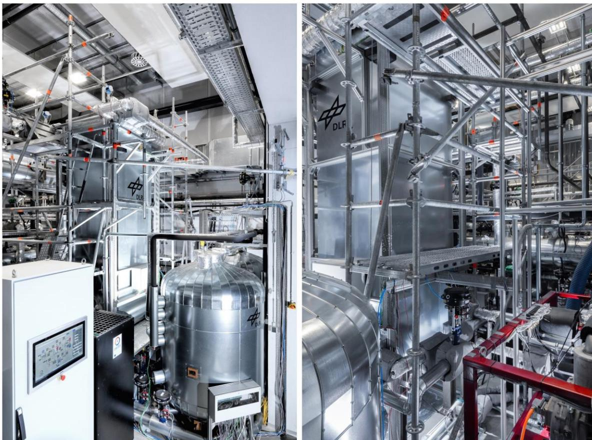
Figure 25: CHESTER installation at DLR Stuttgart. Heat pump, latent heat and sensible heat thermal energy storage (left) and latent heat thermal energy storage and ORC (right). © DLR (CC BY-NC-ND 3.0).
