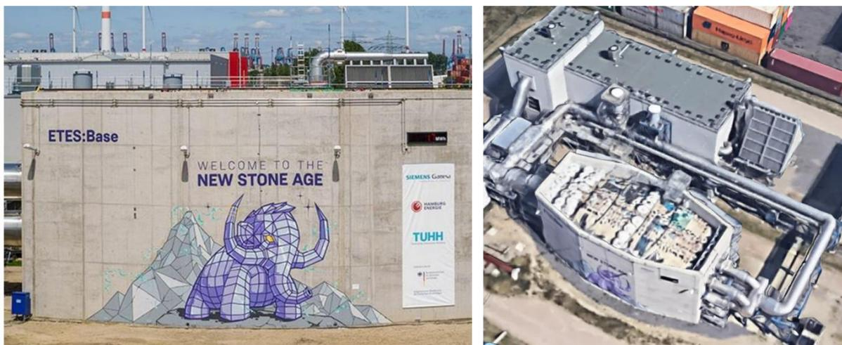
Figure 16: TES: Base System built by Siemens Games in cooperation with TU Hamburg and Hamburg Energy in 2019, source: IEA ES Task 36 Fact-sheets (left) and Google Maps (right).
