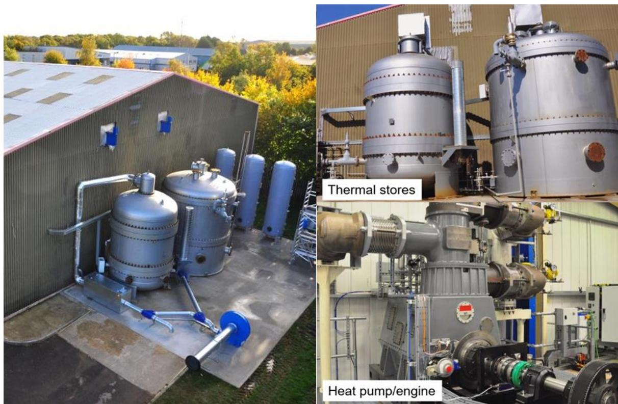
Figure 28: 150 kW Brayton Carnot Battery demonstrator built at Hampshire, UK.
