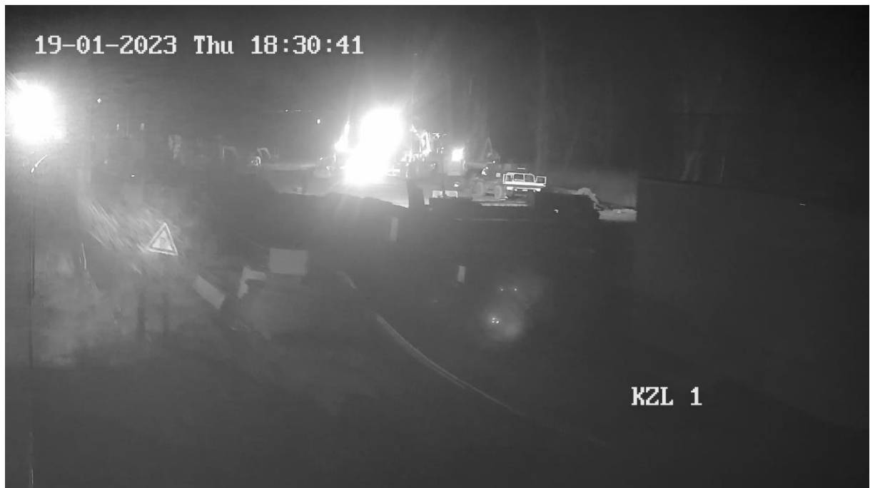
Photograph 6. A general view of the route immediately after clearing the bridge over the Regalica River (a frame from the footage recorded by the rear right mirror camera of the locomotive of train TME 684013)
