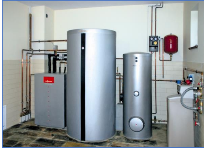
Pic. 6 muratorodom: heat pump installation
