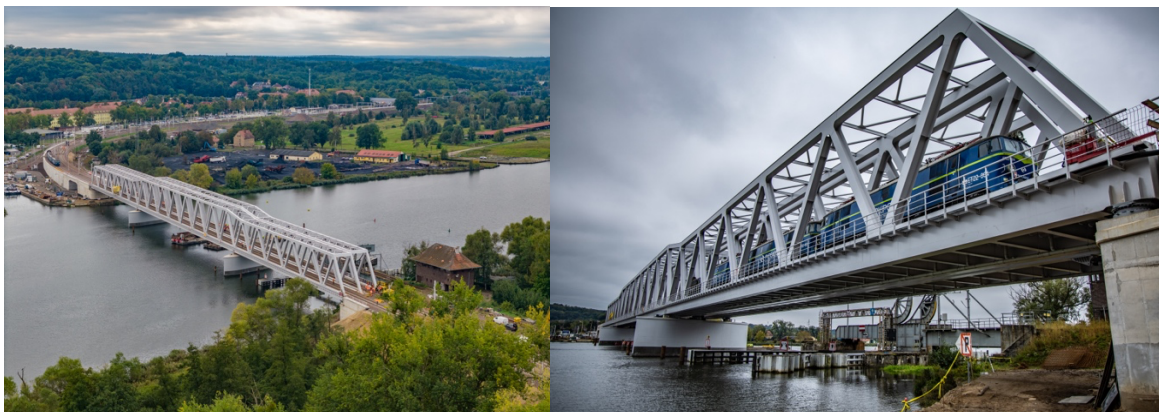
Photo number 1 and number 2: Post-completion photos
