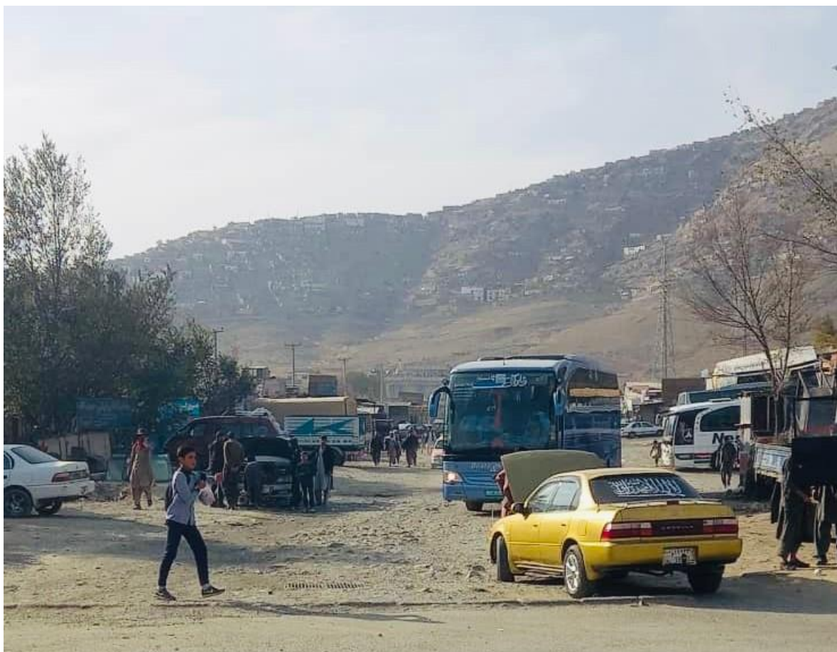
This photograph shows the road infrastructure and one of the bus turning loops in Kabul. Moreover, it is possible to see the slums in the background, at the foot of the mountain. Private archive.
