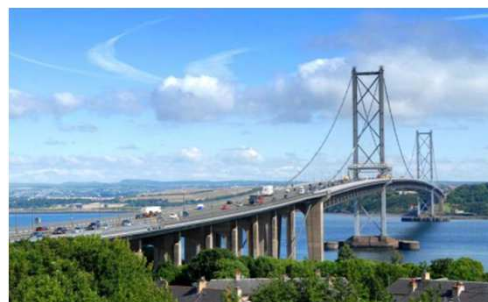
Forth Road Bridge in Scotland
