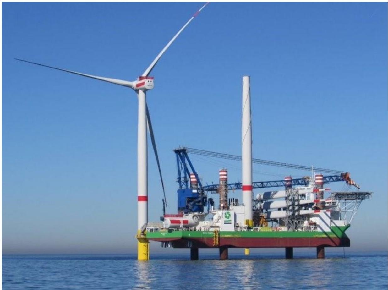
Figure 15. Installation of wind turbines by a jack-up vessel. Source: COWI
