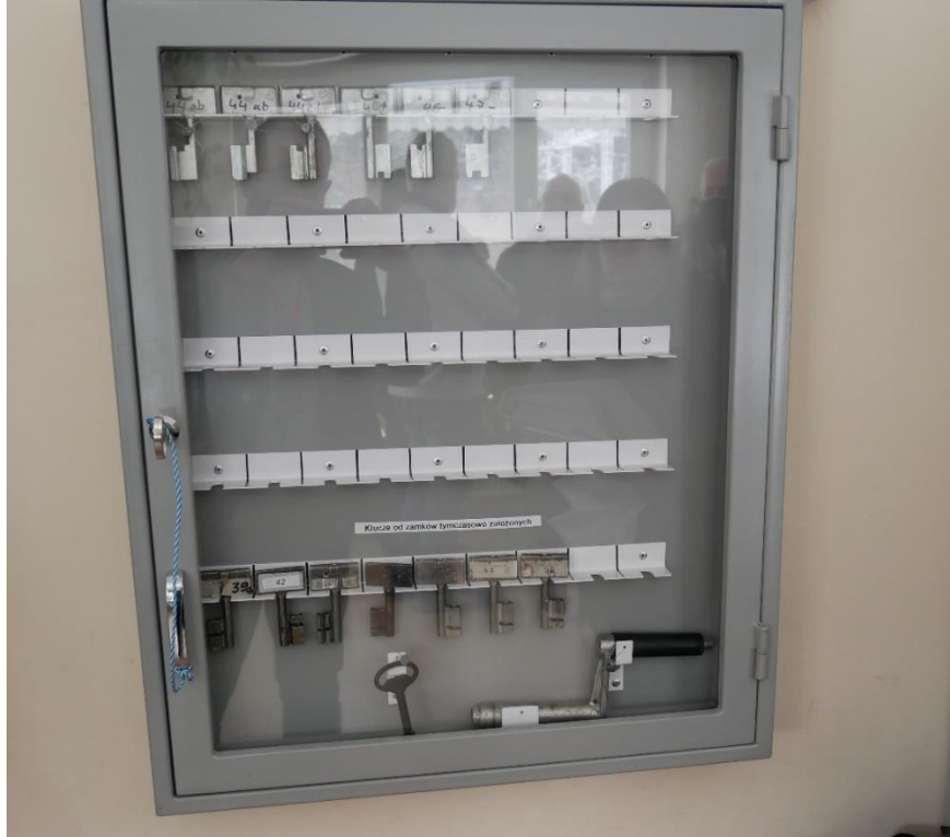
Photograph 4 – Board of spare keys and keys for the locks temporarily installed on the Gg2 signal box
