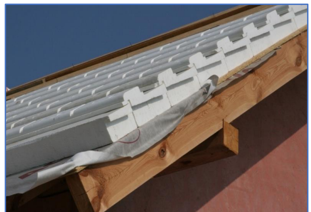
Pic. 1 Lipińscy Domy: polystyrene insulation
