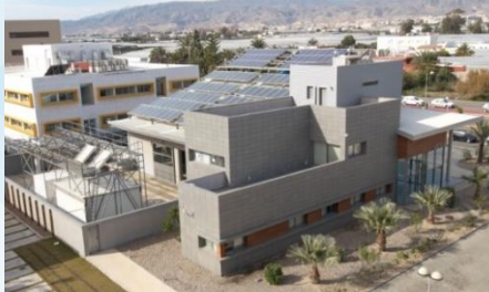
Solar Energy Research Center UAL
