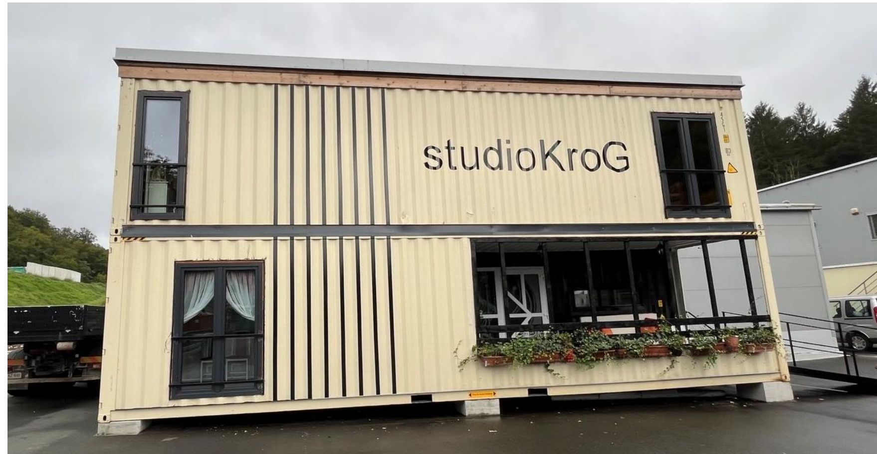
StudioKroG: The first demonstration center of the circular economy in Slovenia on the example of used shipping containers
