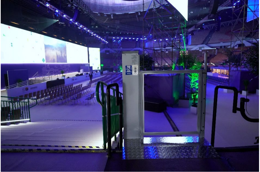
Pic. 4. Vertical hoist installed temporarily for the needs of the WUF11 in the main hall of the Katowice Spodek Arenta, photographed by M Kuświk
