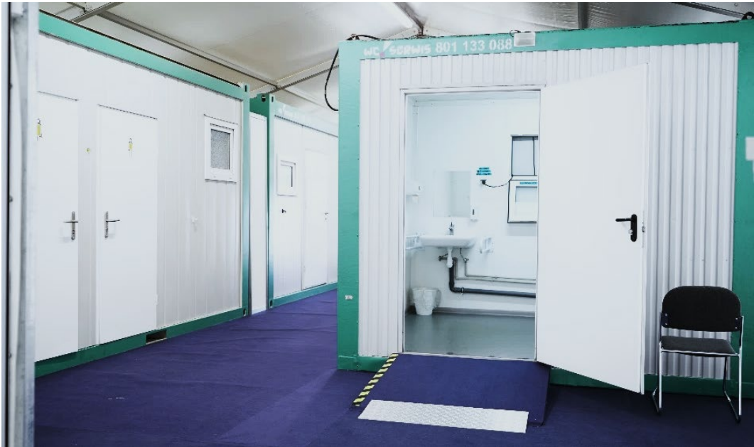
Pic. 7. A container with additional toilets adapted to the needs of people with disabilities placed in one of the tents during the WUF11, photographed by M. Kuświk
