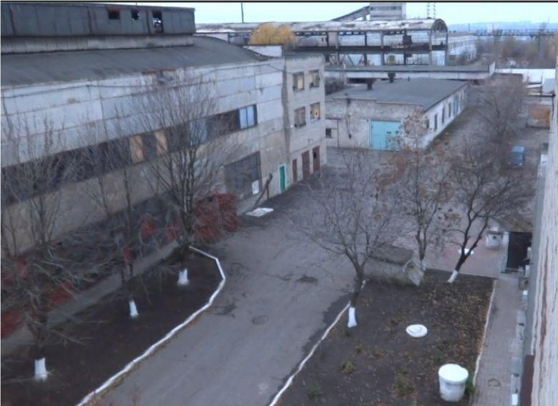
The Plant of Insulating Materials in Donetsk is used as "Izolyatsia" pre-trial detention centre, 3 Svitloho Shliakhu Str., Donetsk, source: https://t.me/traktorist_dn
