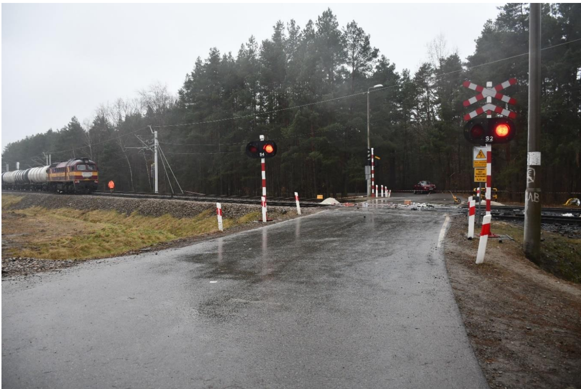
Fig. 9 - View of the crossing from the direction of the van (railway commission material)
