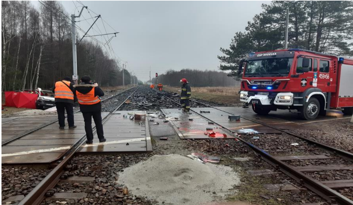
Fig. 4 - The scene of the accident (railway commission material)
