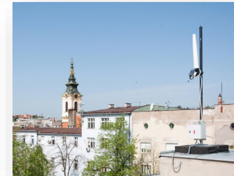
EMF sensor installation
