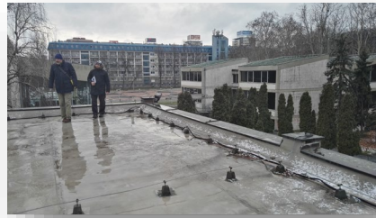
Site visit due to installation
