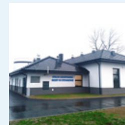
Fig. 13. Water purification plant in Stefanów k. Jarocina, photo by PWiK in Jarocin
