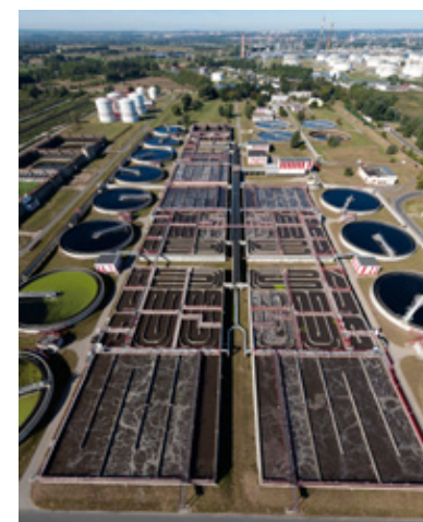
Fig. 11. Wschód Gdańsk Sewage Treatment Plant Photo by GIWK Sp. z o.o. and aeromedia.pl
