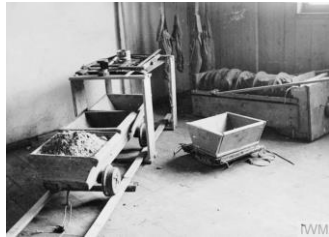
A cart used to remove the earth and a device for pumping air into escape tunnels, both made by POWs, in the storage at Stalag Luft III. © IWM (HU 21225)
