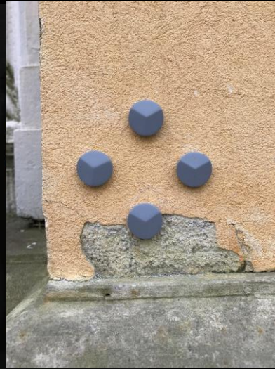
Monitoring of deterioration processes
