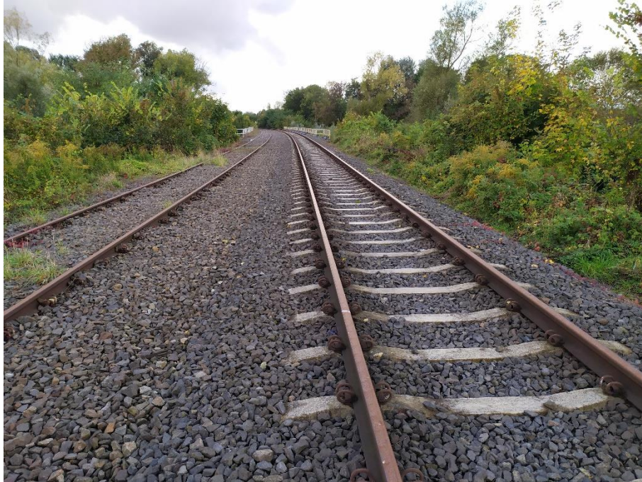
Photo 1. Track in the central part of the Task prior to the start of works.
