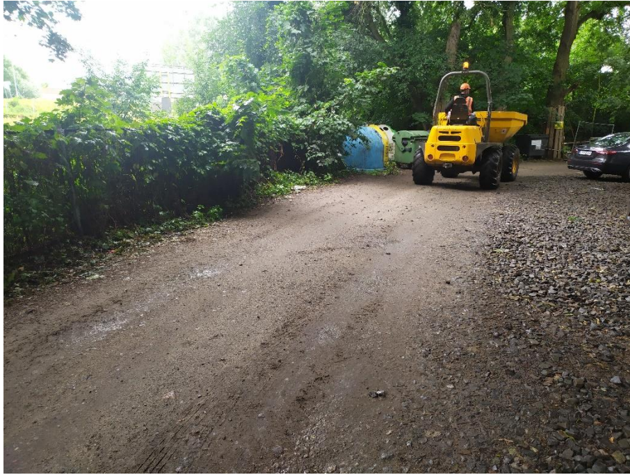
Photo 11. Inspection of the condition of access roads.
