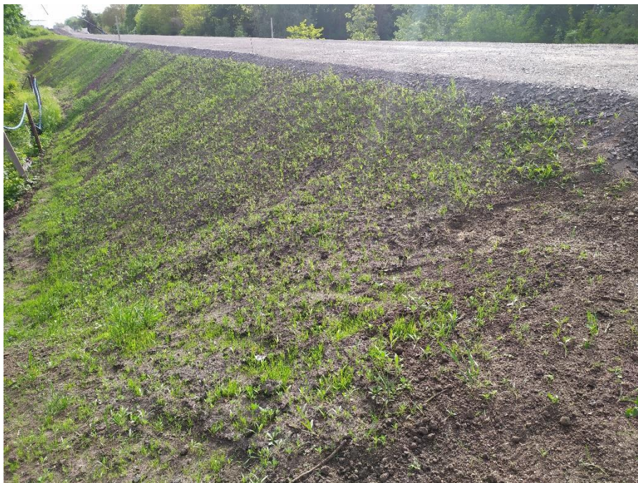
Photo 12. Railway embankment – land reclamation.
