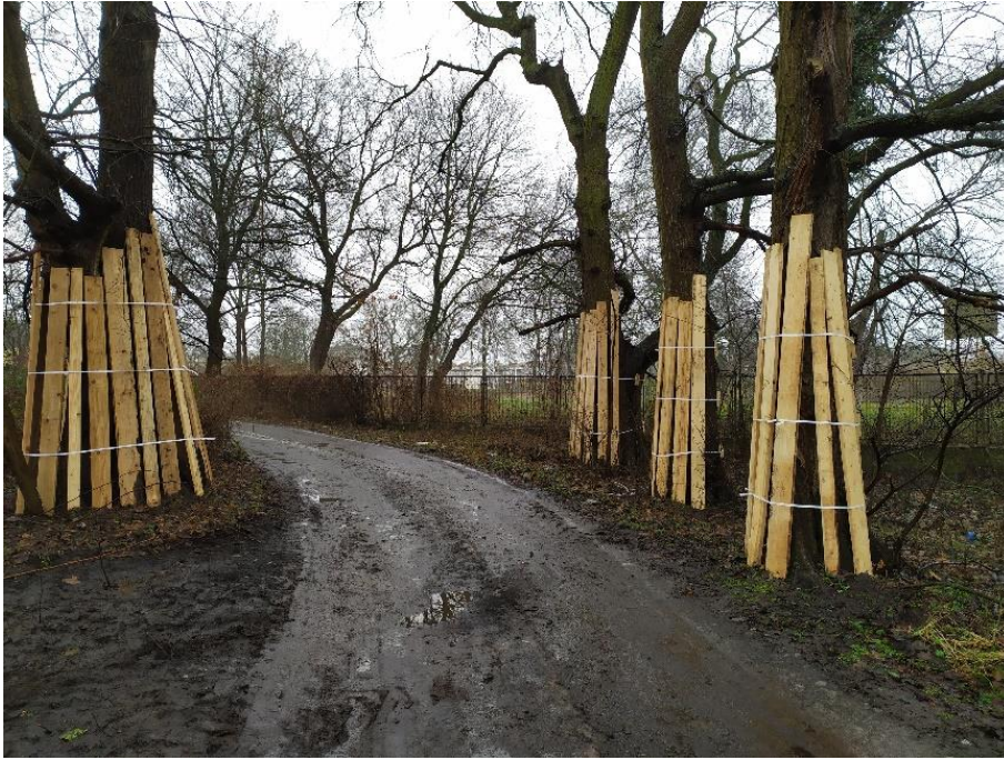
Photo 3. Protection for trees at risk of damage.
