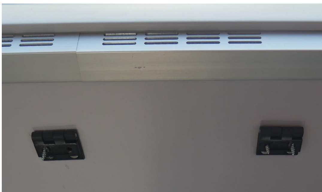
Photo 4 – fixing system of the table (photo by PKBWK)
