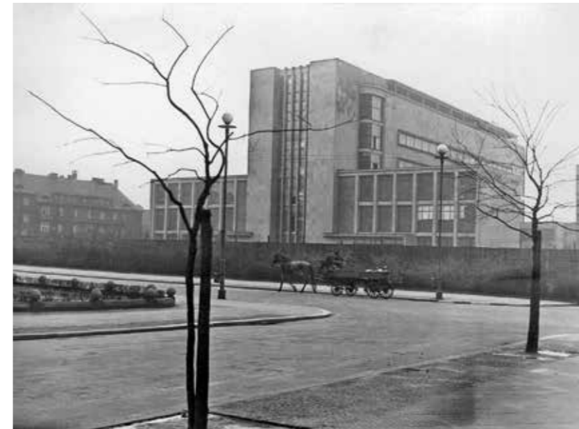
Photo 5.2. The Muzeum Śląskie (Silesian Museum) building, completed in 1939. One of the principal state-of-the-art buildings in pre-war Poland, with photocells on its front entrance, escalators, air conditioning, and a convection central heating system (The Silesian Library Collections, Special Collections Department)
