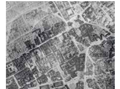
Left: Photo 9.1. Warsaw. Aerial photograph (ortho-photo map detail), June 1945. The empty white space on the left is the area of the Warsaw Ghetto, which the Germans demolished in 1943-1944. The rest of the built-up area was devastated during the Warsaw Uprising of 1944 (Collections of the State Archive in Warsaw)
