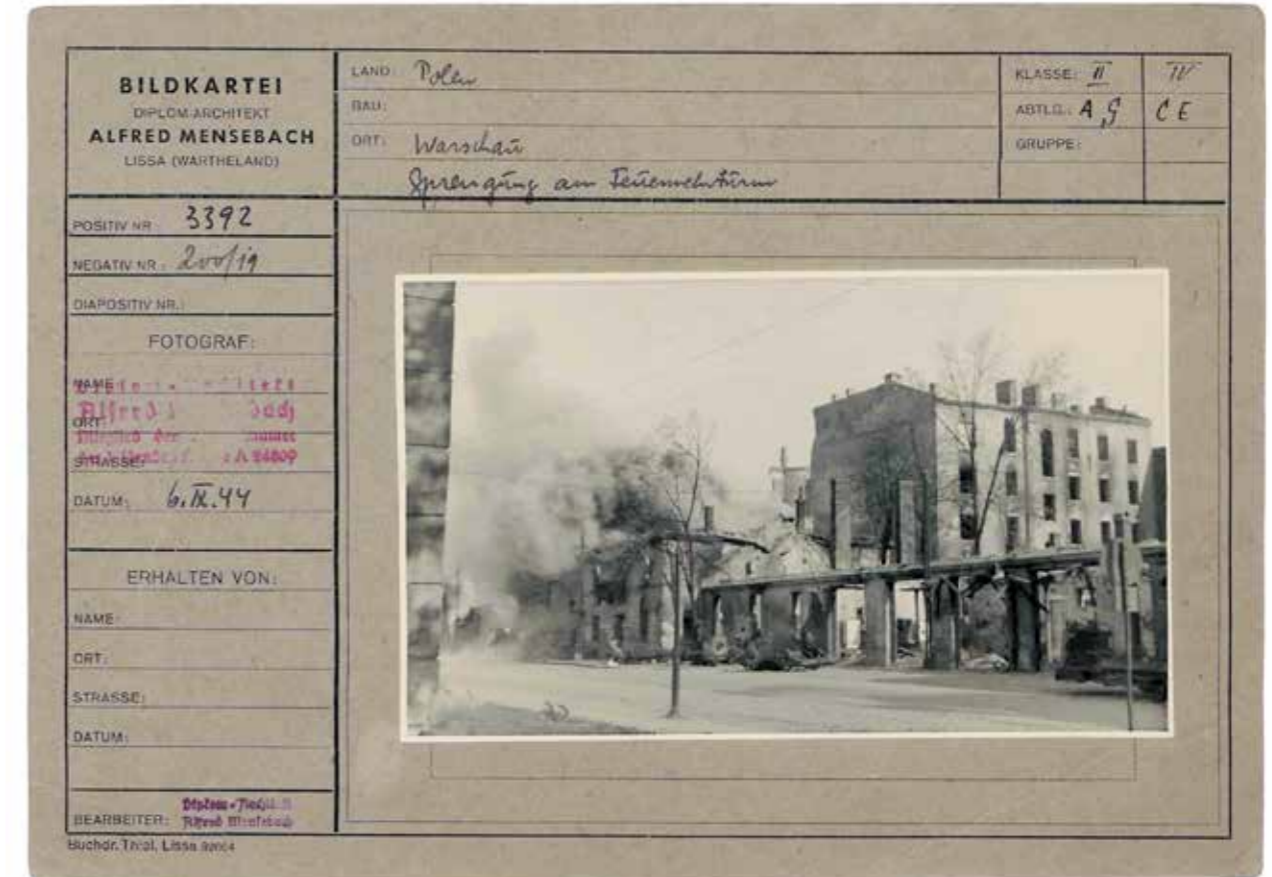
Photo 8. Sprengung am Feuerwehrturn, 6.IX.44 [Blowing up the fire station tower, 6 September 1944]
