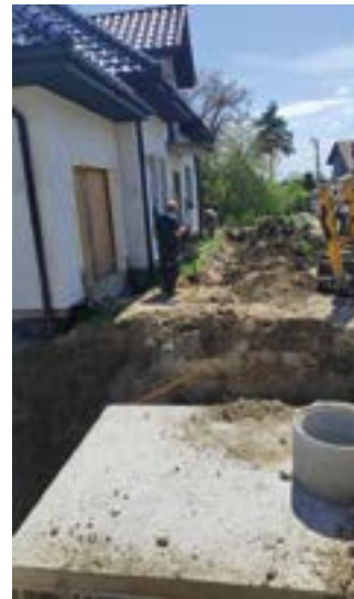
■ Assembly of a rainwater retention and purification system for a single-family building in Bieruń by contractor AquaSmart from Krakow
