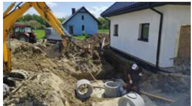
■ Assembly of a rainwater retention and purification system for a single-family building in Bieruń by contractor AquaSmart from Krakow
