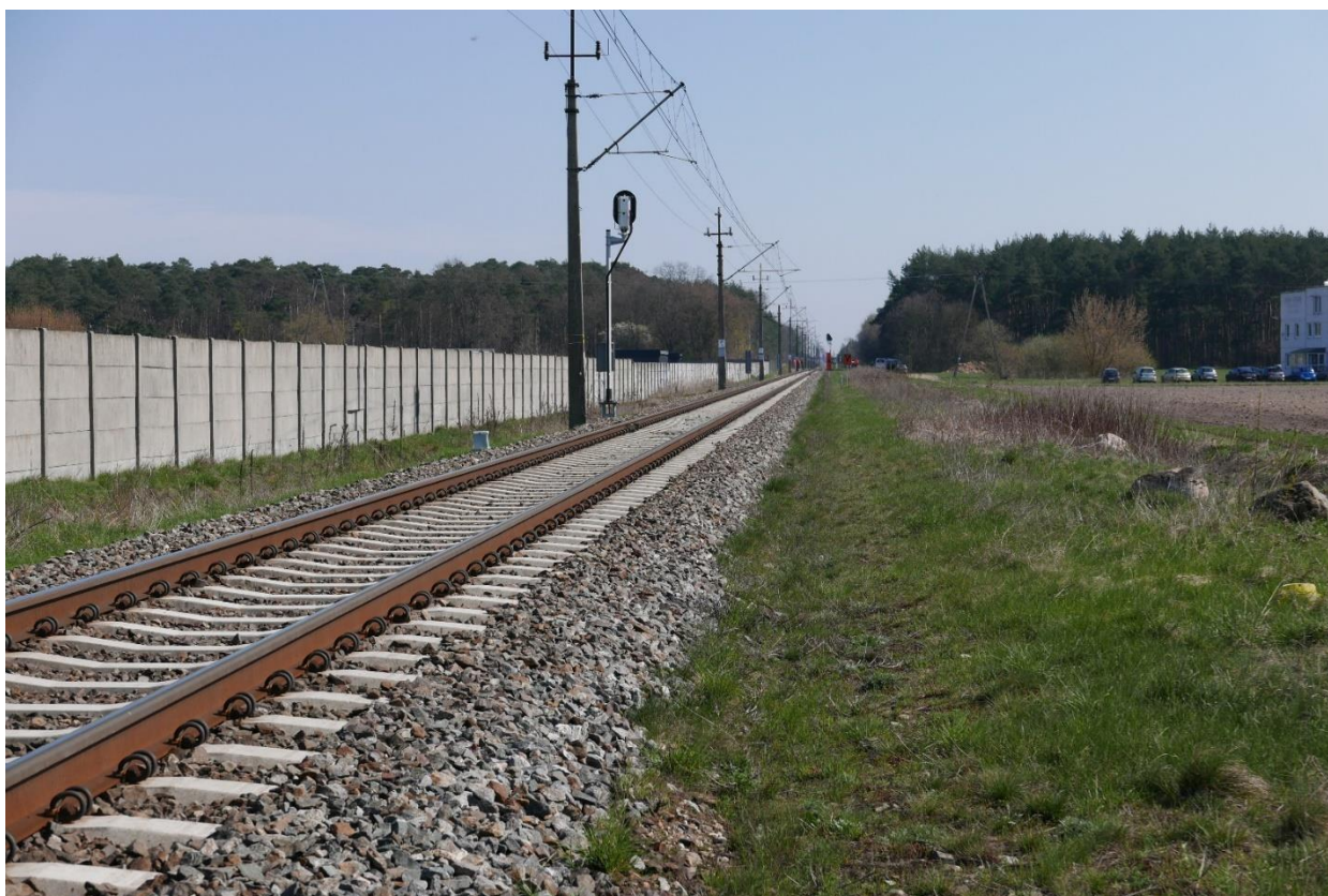
Photo 7. Fence and traction poles restricting visibility (source: GDPWK)
