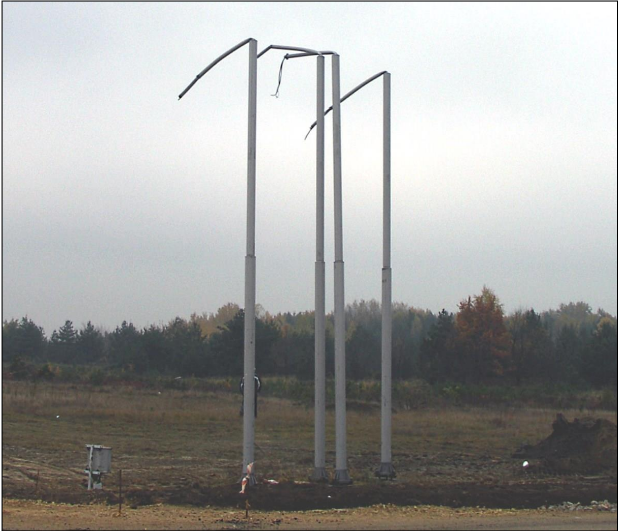
11 – Damage to the approach lights system ahead of EPKT RWY27 threshold after the accident
