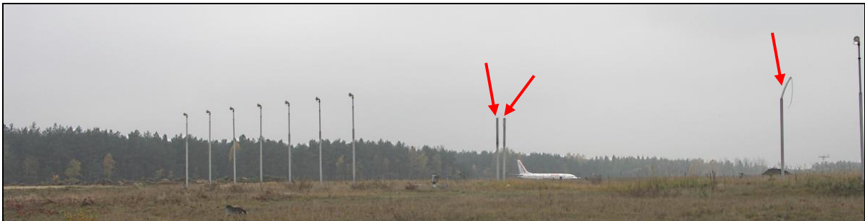
16 – Damage to the approach lights system ahead of EPKT RWY27 threshold after the accident
