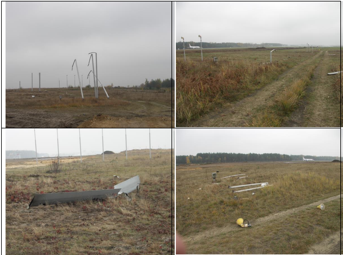
Fig. 7-10. Damage to the approach lights on EPKT
