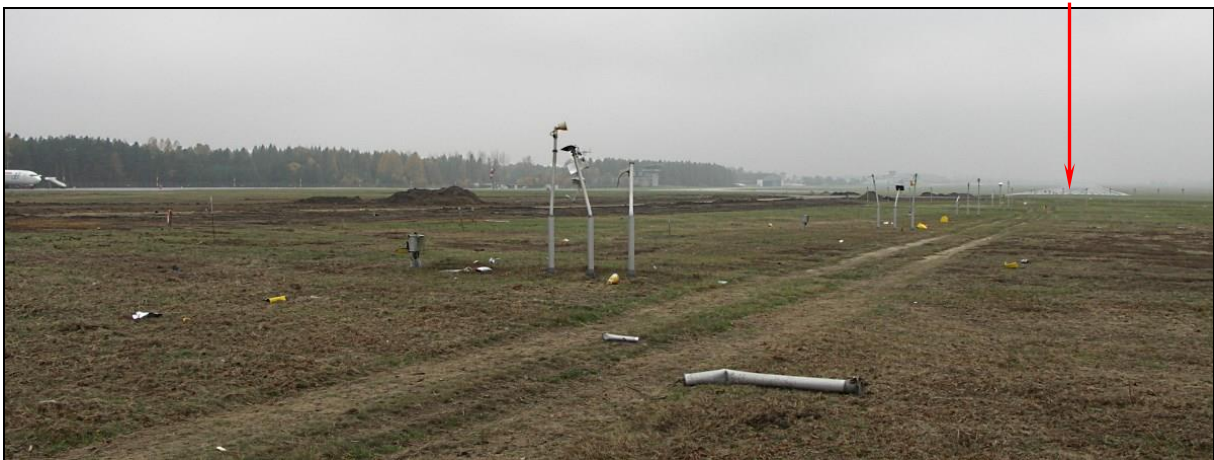
23 – Damage to the approach lights system and small pieces of the airplane skin. Visible RWY27 threshold
