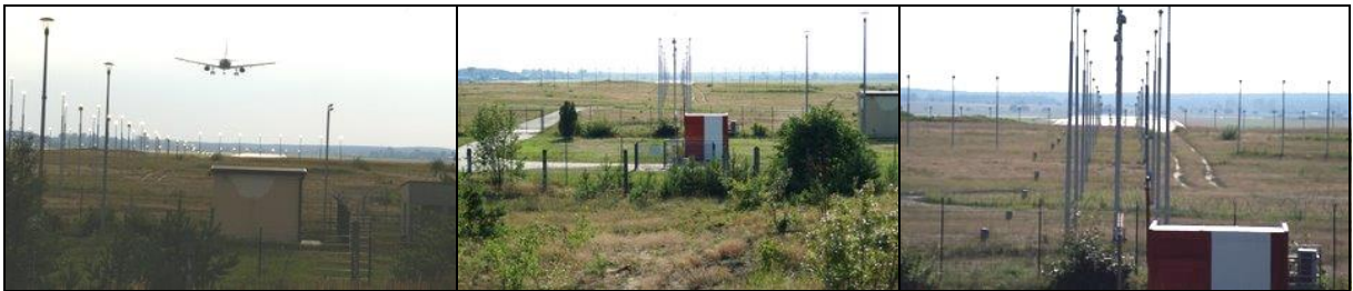
6, 7, 8 – Approach lights situated ahead of EPKT RWY27 – condition prior to the accident [photo: internet site publicly available]
