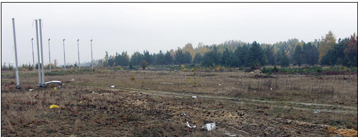
12 – Damage to the approach lights system ahead of EPKT RWY27 threshold after the accident
