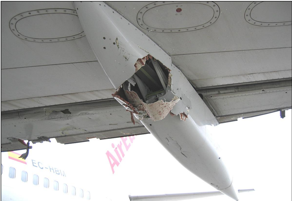
62 – Damage to the track fairing of the left outboard flap; visible damage to the flap [photo: airplane crew]
