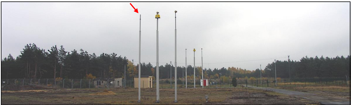
9 – Beginning of the approach lights system ahead of EPKT RWY27 threshold after the accident
